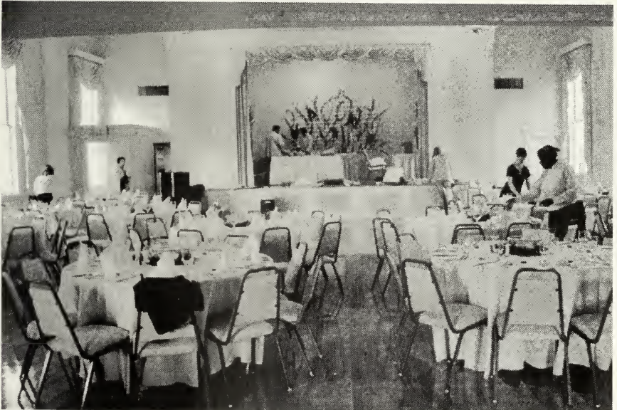
Upstairs in former Parish House after its conversion to Topsfield Commons
